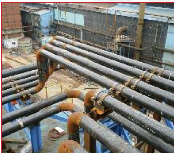
Preinstallation of pipework
