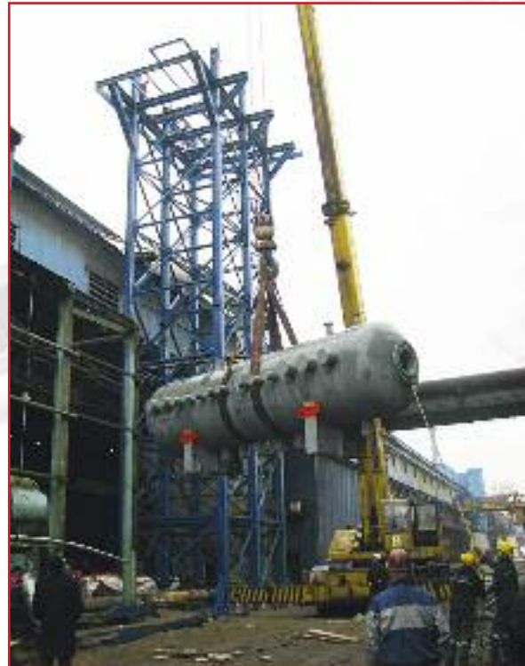
Installation of the steam drum
