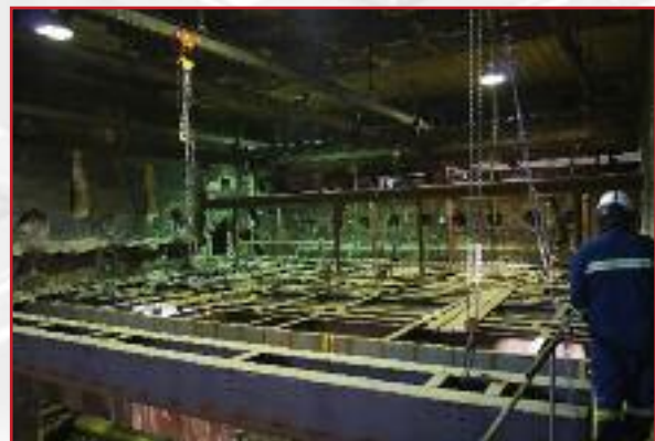
Skid system installation
